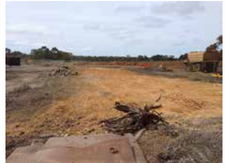
Workshops & Tanks zone
