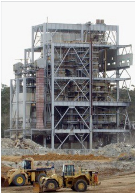
The remaining power station structure.
