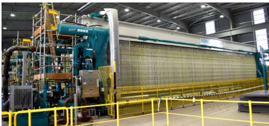
Figure A: Kwinana Refinery Residue Filtration Facility.
