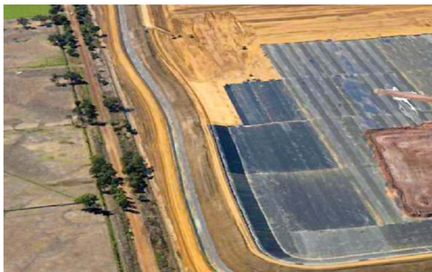
Figure 7-4: Contouring external residue embankment trial.
